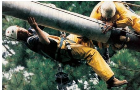
Denso Steelcoat™ System applied in-situ to protect aerial pipelines, New Zealand.
