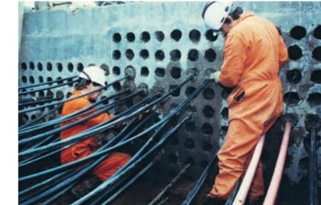
Electrical cable duct entries at UK ethylene plant, sealed with Denso Mastic.
