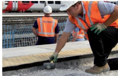
Concrete to asphalt platform joints sealed with the Denso Road System, UK.
