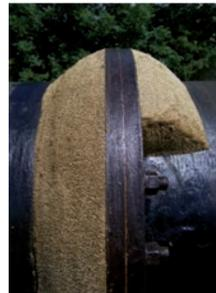
Application of Denso Profiling Mastic™ to a pipe flange.
