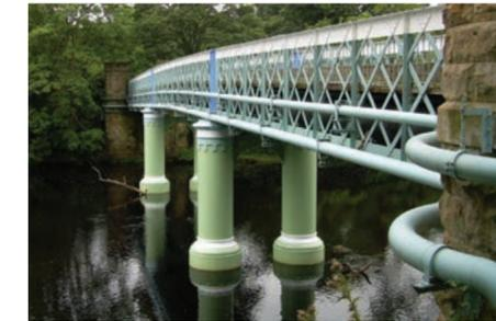
Water pipe bridge, UK, protected with Denso Steelcoat™ System, applied in-situ without grit blasting.
