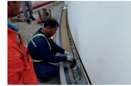
Application of Denso Steelcoat™ Tank Base Protection System, UAE.
