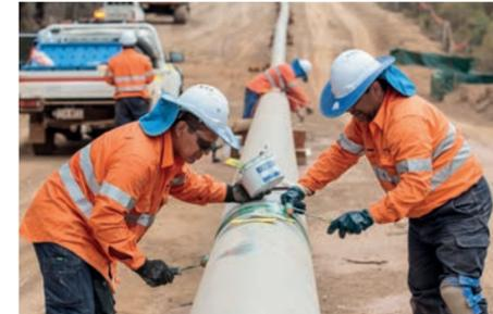
Denso Protal applied to Field Joints, Australia.
