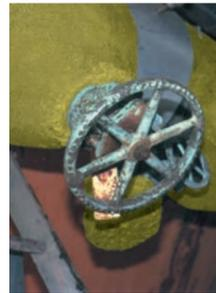
Application of Densofil™ to insulate and protect a valve.
