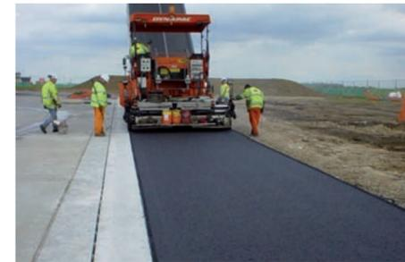
Runway re-surfacing, UK, mastic asphalt joints sealed with Denso Road System.
