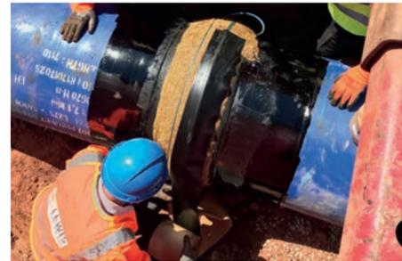
Application of Denso P2 Joint Protection System to water pipeline, UK.
