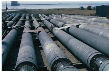
Subsea joints of sea-outfall, Atlantic Ocean, protected with DensoPol™ Marine Tape System.
