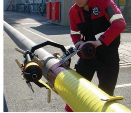
Application of two Denso tapes simultaneously using a Denso wrapping machine.
