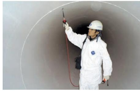
Denso Archco™ Liquid Reinforced System protects a tank's internal surfaces, Korea.
