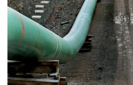
The welded joint areas on this North American pipeline are protected with a Denso Protal™ Liquid System.
