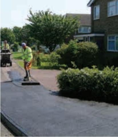
Sprayco K3-60 is a slow breaking cationic bitumen emulsion designed to be used as a slurry seal binder and complies with the requirements of BS 434 part 1. Sprayco K3-60 is classified according to BS EN 13808:2013 as a C60B5 bitumen emulsion. Seasonal grades are available.
