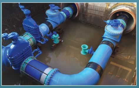
FT Pipeline Systems can manufacture all the fittings for your scheme. CAD drawings are provided in consultation with the client and are agreed upon prior to the start of manufacturing. Standard fittings are produced according to BS EN 10224. Alternatively, bespoke fittings can be manufactured to suit specific requirements.
