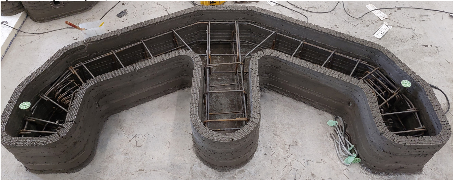
Fig. 4: reinforcement within the printed perimeter
