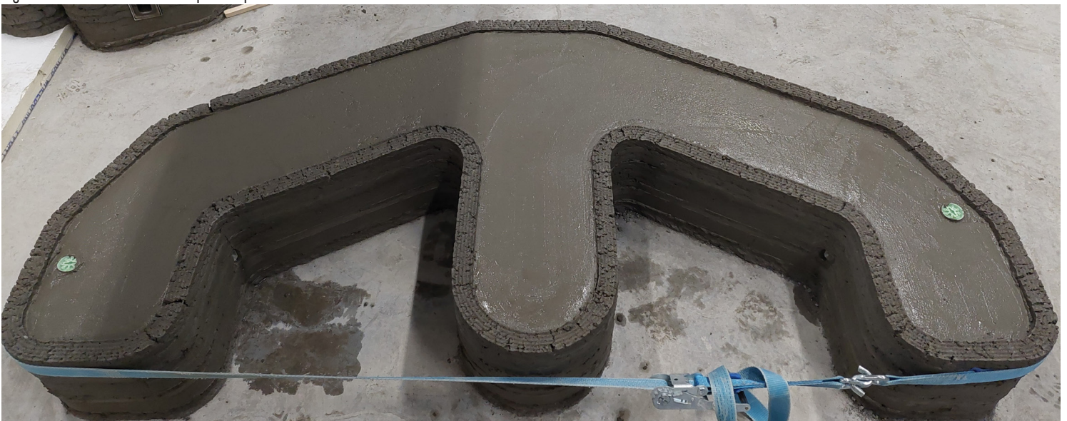
Fig. 5: concrete poured within the permanent formwork
