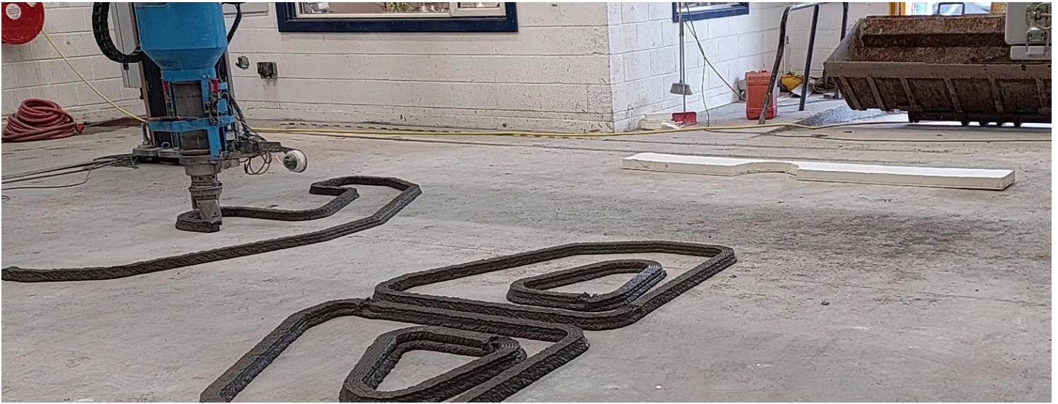
Fig. 3: demonstrating the printing of the perimeter
