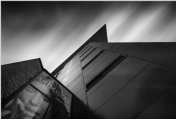
Above: Cardiff and Vale College near the Bay in Cardiff
