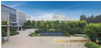
Shijiazhuang Enric Gas Equipment
