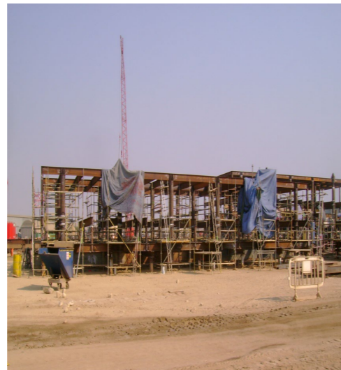
Central piperack / 6 piperack structural sections (750 mt)
