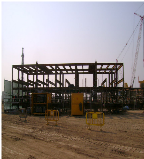
Central piperack / 6 piperack structural sections (750 mt)
