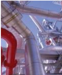
Pipeline & Process Services
