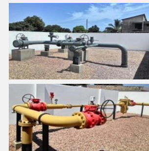
Pigging Launcher and Metering
