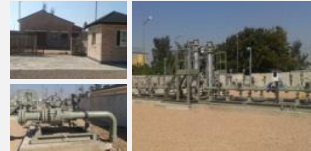
IRS (Intermediate Regulation Station) and Pigging Receiver
