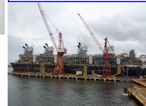
FLNG : On site: Q2- 2024
