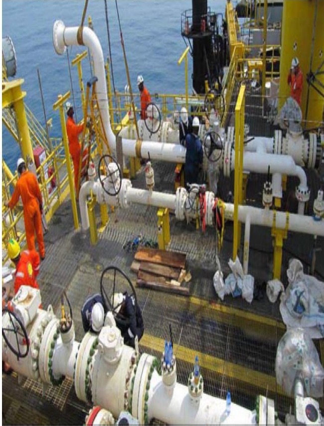
Assembly of 12-Inch S. Forcados Line on Sea Eagle
