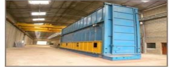
Fabrication/Galvanizing Facility, Oko-Oba, Agege - Lagos
