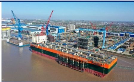
FPSO : Moving to site
