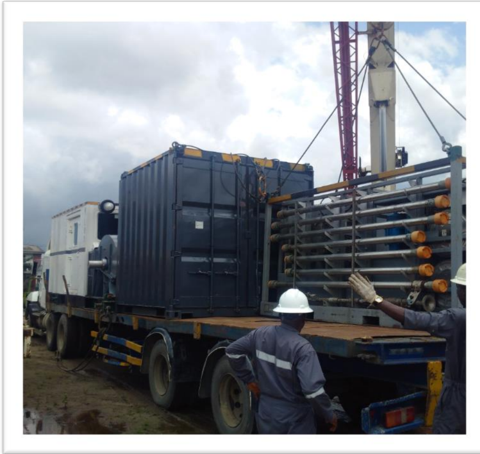
Equip Loadout with Pressure Control Equipment
