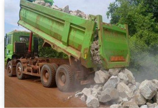
Rockfill delivery to access route
