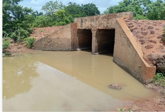
Existing crossings surveyed
