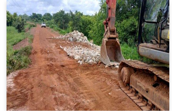
Road formation and shaping
