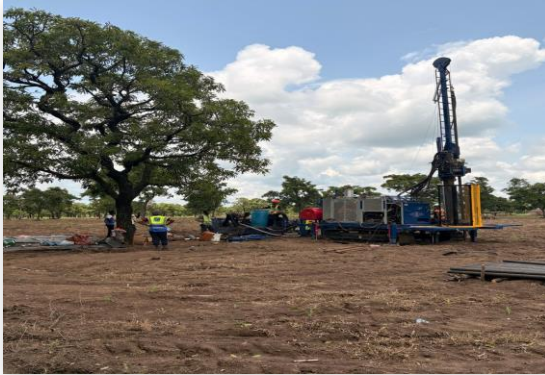
Geotechnical drilling at the well site
