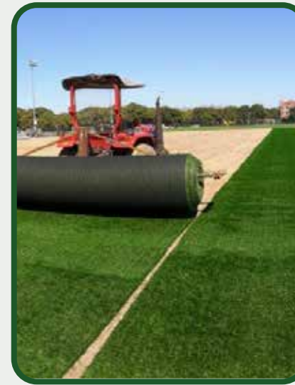
LAYING OF ARTIFICIAL MATRIX
