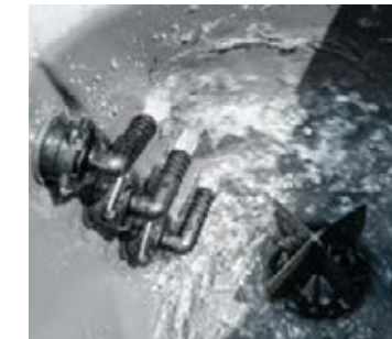
High-performance diffusers on the wall and on the overflow optimise induction.
