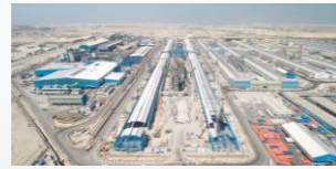
EPC Alba Aluminium in Bahrain. One of the world's largest aluminum smelter facilities, incorporating 5km of electrolyzer modules
