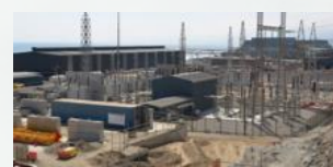
Green ammonia tank in the UK. Best available technology study and FEED for 1x low temp 80,000m3 storage tank
