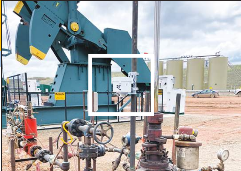
MethaneTrack™ endpoint mounted in close proximity to pump jack & well head
