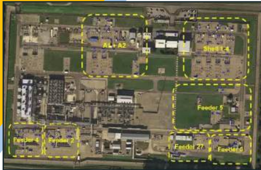
Installation of 155 MethaneTrack™ endpoints in just 3 days
