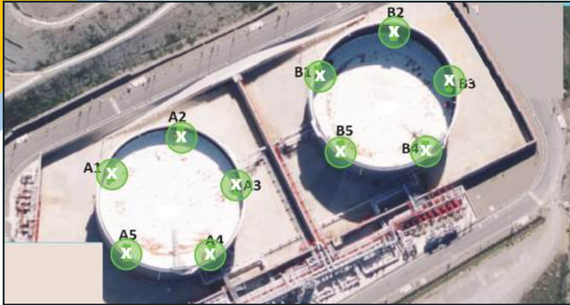
Installation of 10 MethaneTrack™ endpoints in just a few hours
