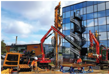
The drill site.
