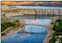
Other renewables such as wind and solar are variable, and hydropower, particularly pumped storage hydropower (PSH), can pick up the slack when they are not producing power. PSH involves a dam with two reservoirs, an upper and a lower one, and a turbine. It can store energy by pumping water into the upper reservoir; when the energy is needed, the water will be released...
