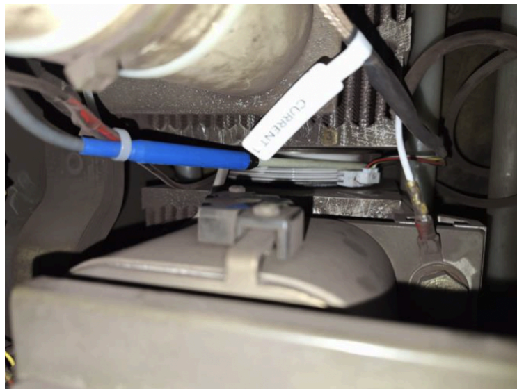
Figure 1 Microwire current sensor on thyristor
