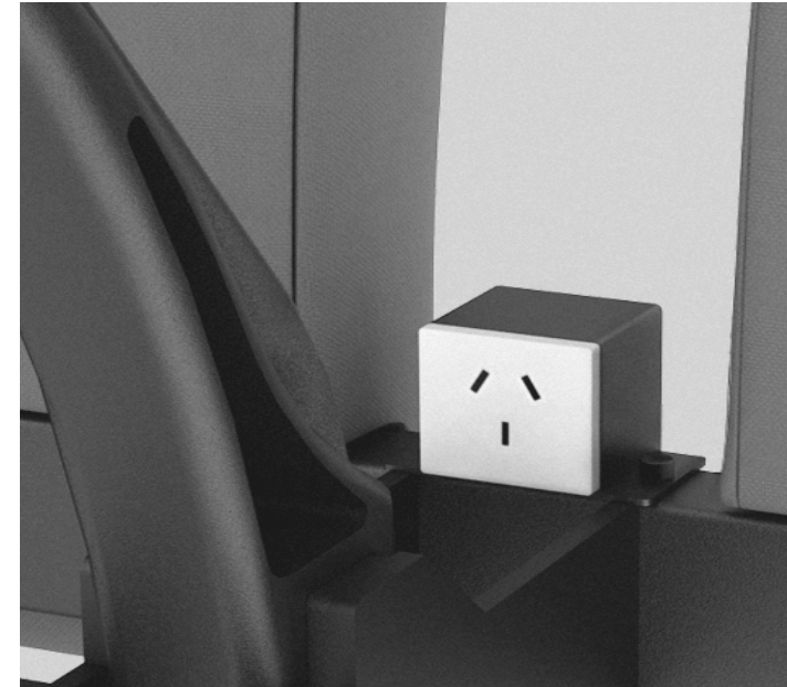
GPO on beam
