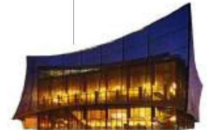
Alhi Grand Theatre Construction 2014
