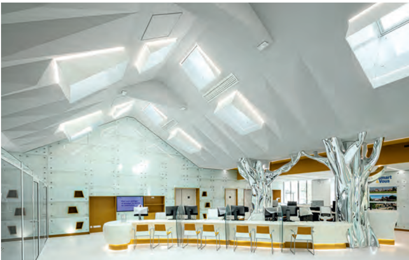
Reception area of the Clamart town hall south-west of Paris. Architects: Bigeault-Taib & Associates, 2020. Vibrasto cladding on the ceiling.
