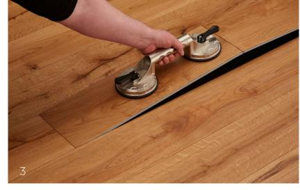
Each plank consists of an Oak surface layer and engineered core, the magnetised and foam-sealed wood boards provide a secure connection to the supporting pedestal which can be conveniently disconnected using a suction lifter for enhanced access.
