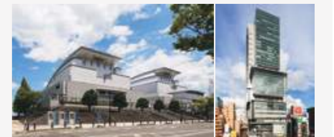
Biwako Hall Center for the Performing Arts Shiga, 1998
