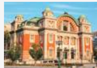
Osaka City Central Public Hall, 1918
