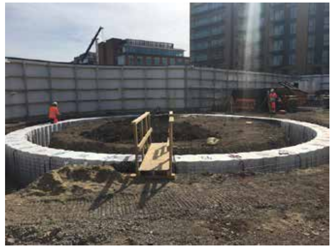
Thames Tideway Project, London
