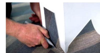
6. With the material now lying flat around the fittings and corners, the final cutting along the wall lengths can be carried out.
