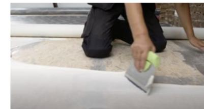
2. Apply the adhesive to the subfloor in accordance with the adhesive manufacturer's instructions.
