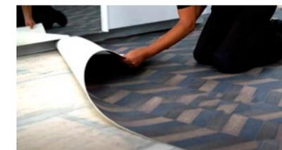
3. Allow the recommended drying time and then reposition the flooring material over the prepared subfloor.
