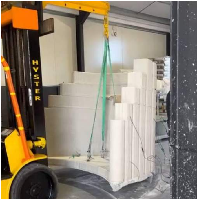
Embedded lifting eyelets
