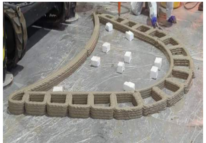
Internal ribs showing the tying of two different walls.
