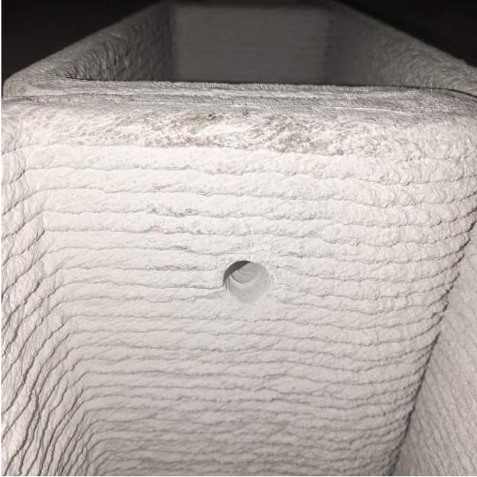
Drilled hole for rebar
