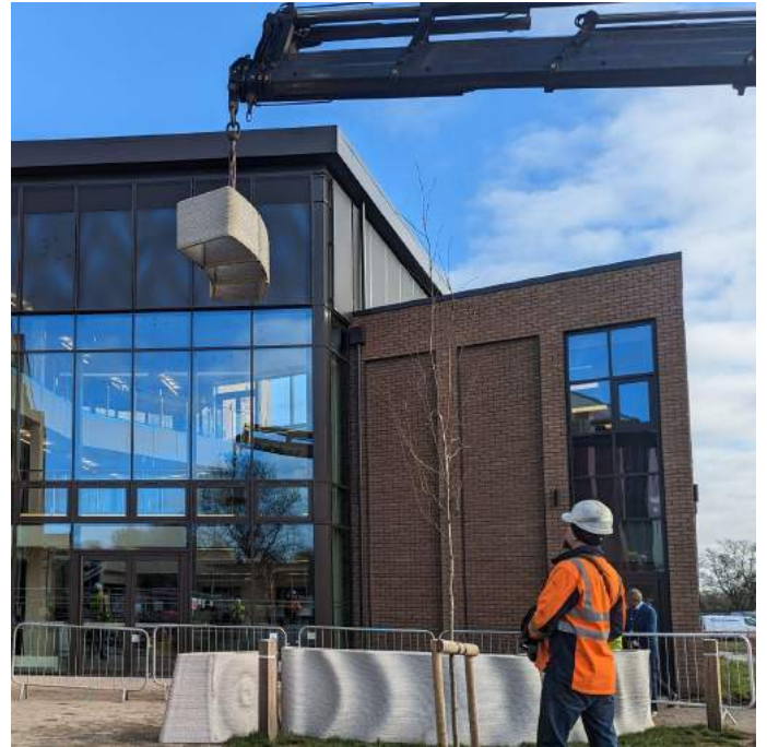
Lifting from internal ribs
