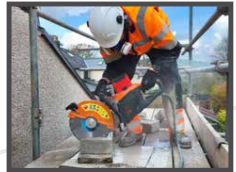
IDEAL FOR USE ON SCAFFOLDING
