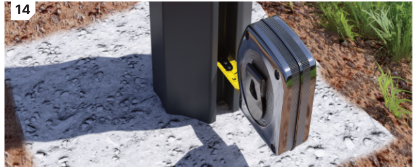
14: When finishing your fence, the distance between your second last and last post might be less than 1.8m.
