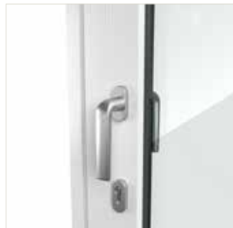
Lockable tilt-and-turn door with window handle
