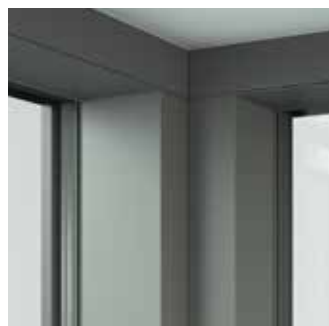
Standard corner coupling, interior
