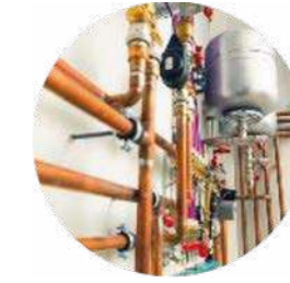
Heating systems filling
