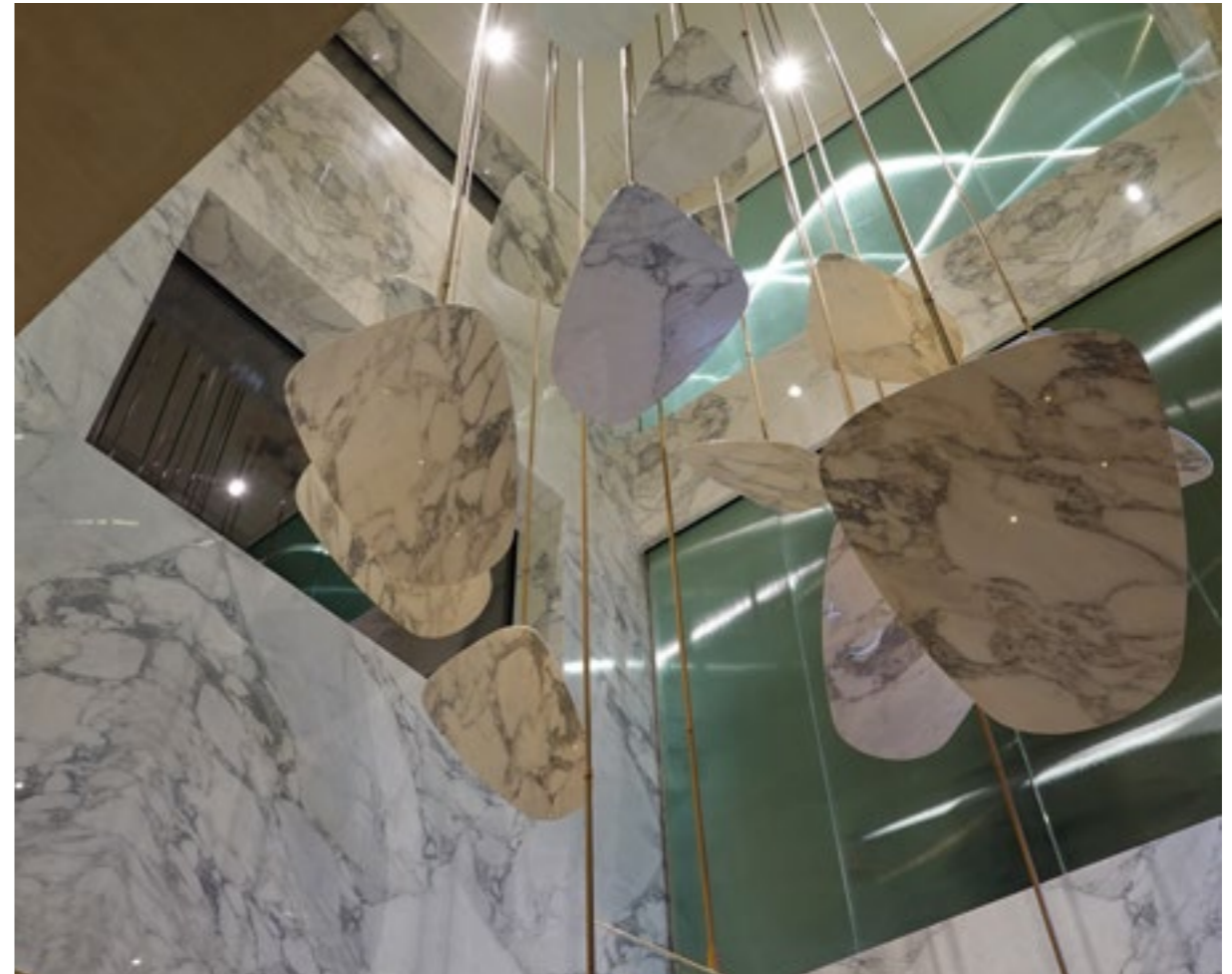
CUT-TO-SIZE LIGHTING INSTALLATION USING 6MM SLABS (FIG.6.1)
