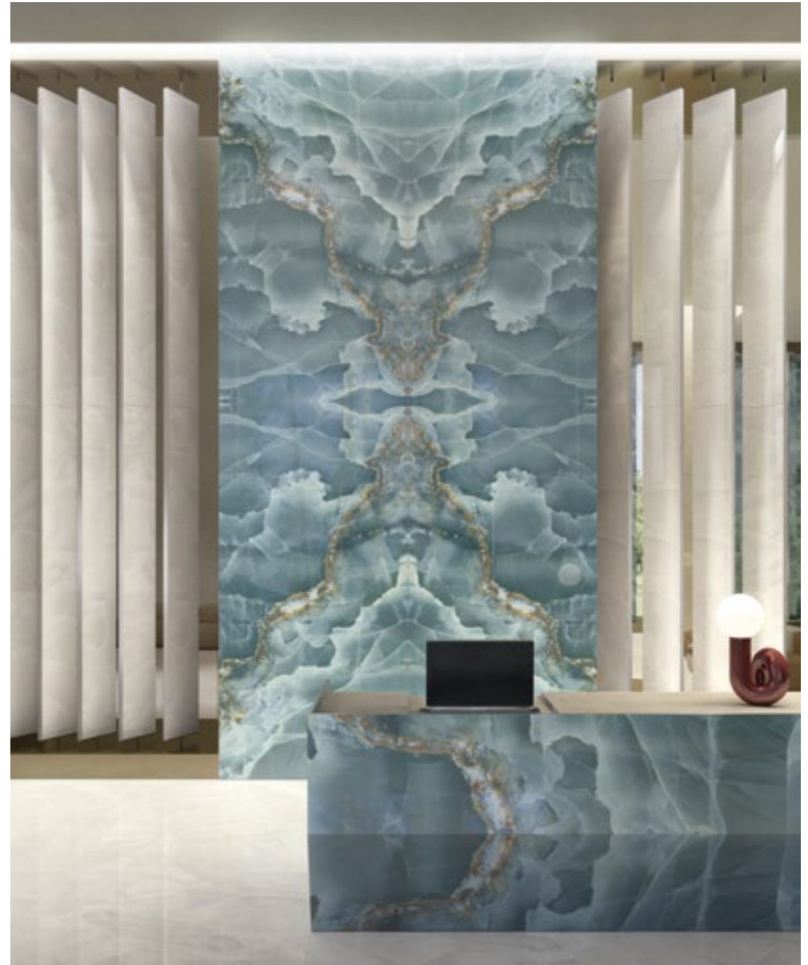
SEAMLESS PRECISION: BOOKMATCHED SLABS TRIMMED FOR FLAWLESS PATTERN ALIGNMENT (FIG.9.1)
