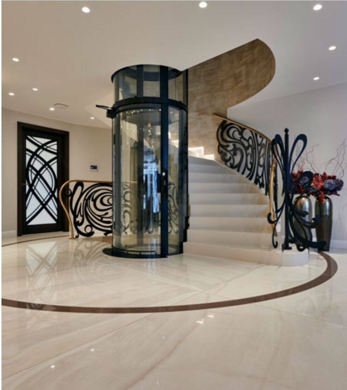
LARGE FORMAT INLAID FLOOR USING 3000 x 1500 mm SLABS (FIG.20.1)
