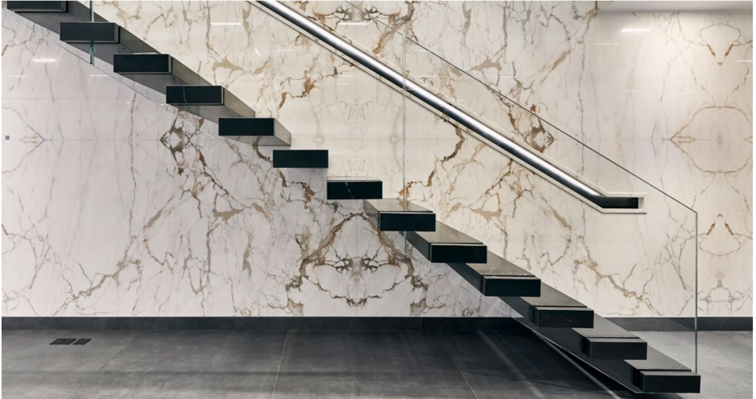
SUSPENDED ELEGANCE: CANTILEVER STAIRCASE WITH PORCELAIN TREADS (FIG.39.1)
