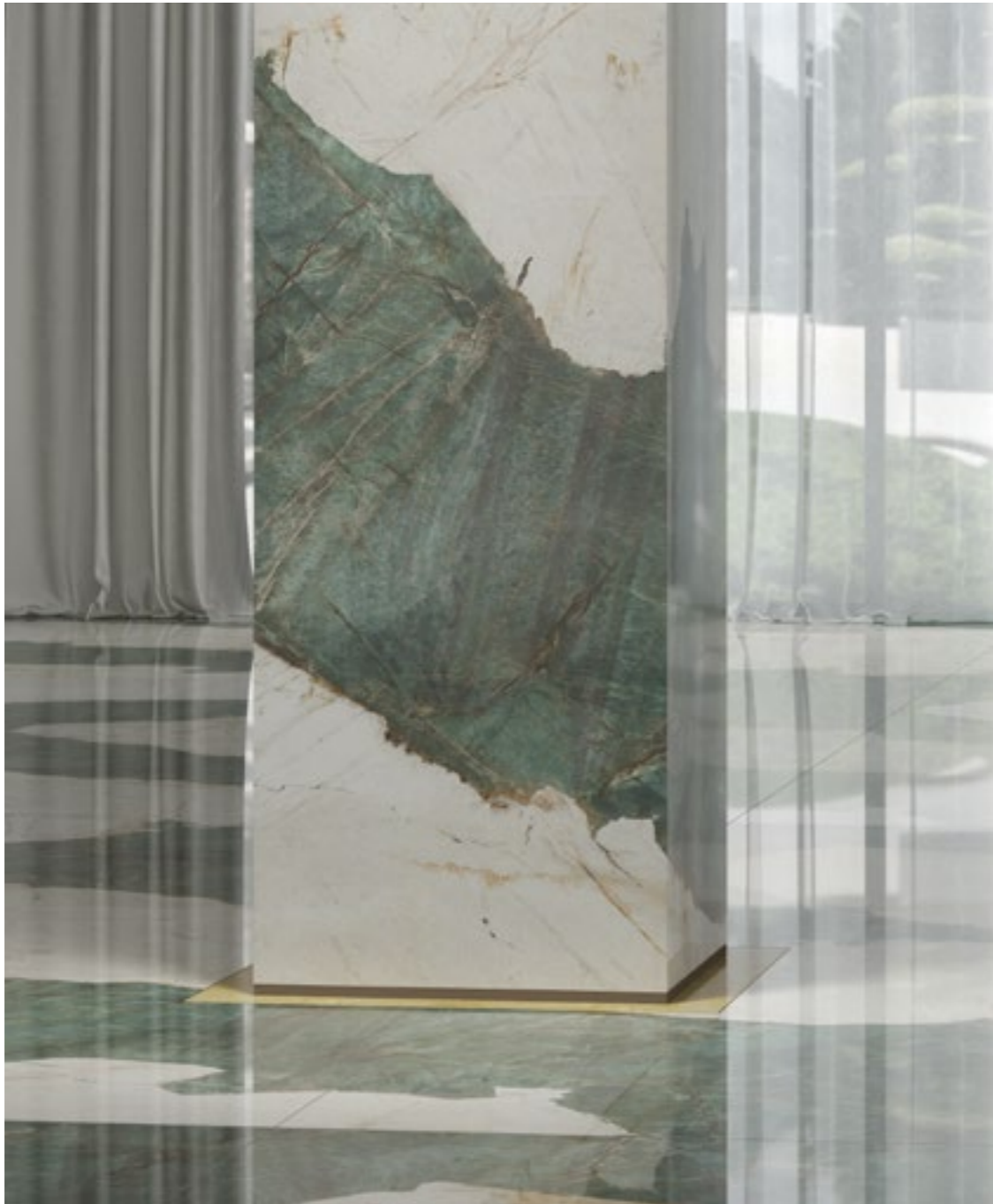
CUT-TO-SIZE VEIN MATCHING PANELS CLADDED OVER RECTANGULAR COLUMN (FIG.13.1)
