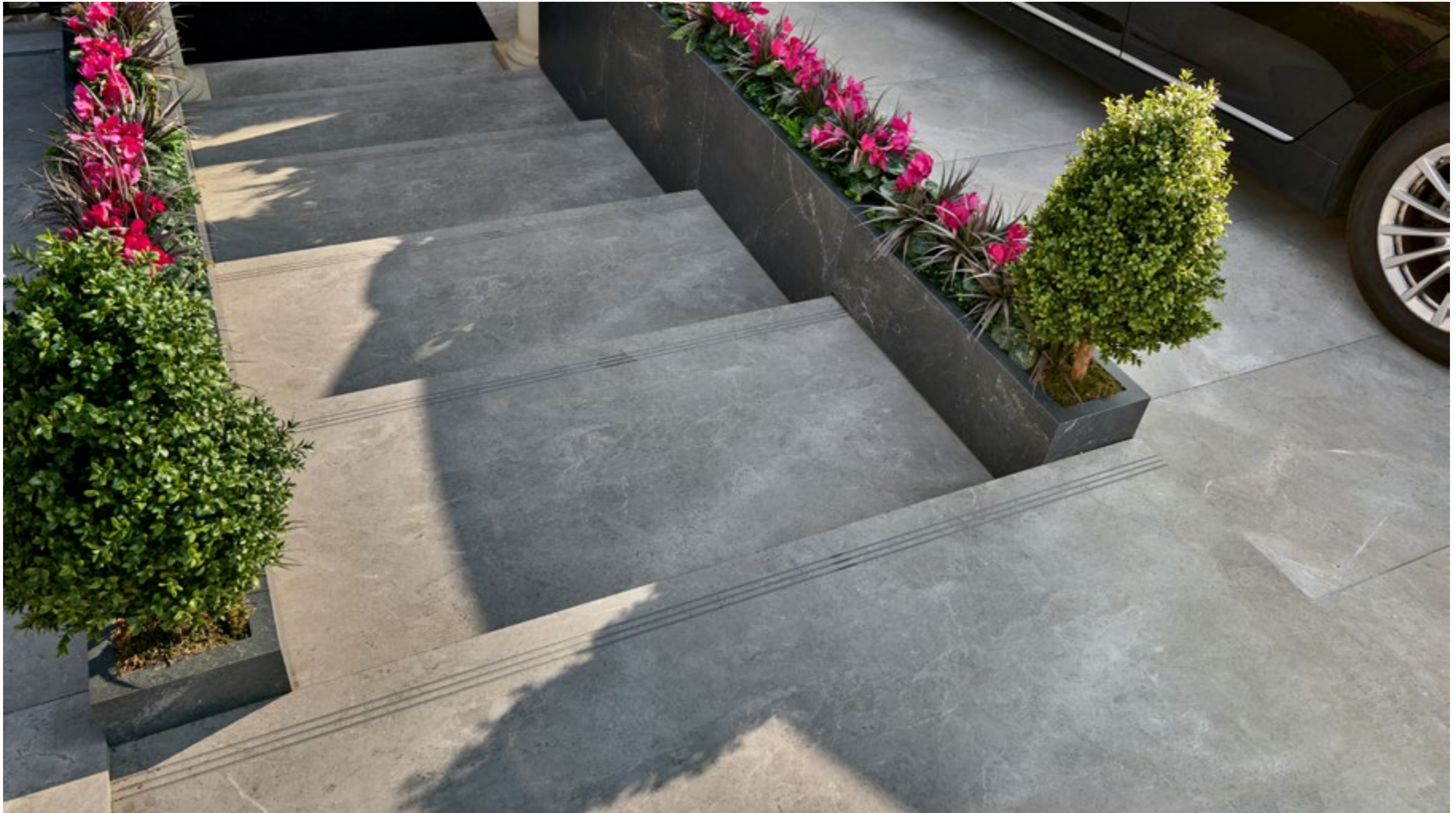
20MM STEPS FEATURING BULLNOSE PROFILE AND ANTI-SLIP GROOVES (FIG.35.1)
