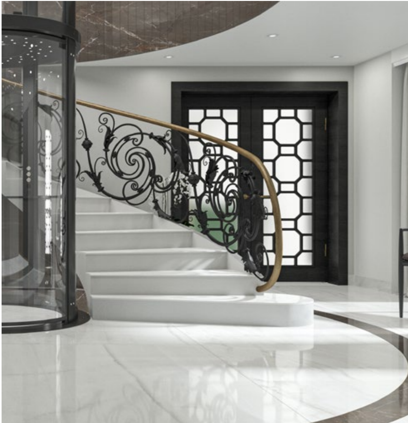
LARGE FORMAT FLOOR SLABS WITH MATCHING 12 MM STEPS WITH BULLNOSE NOSING (FIG.37.1)
