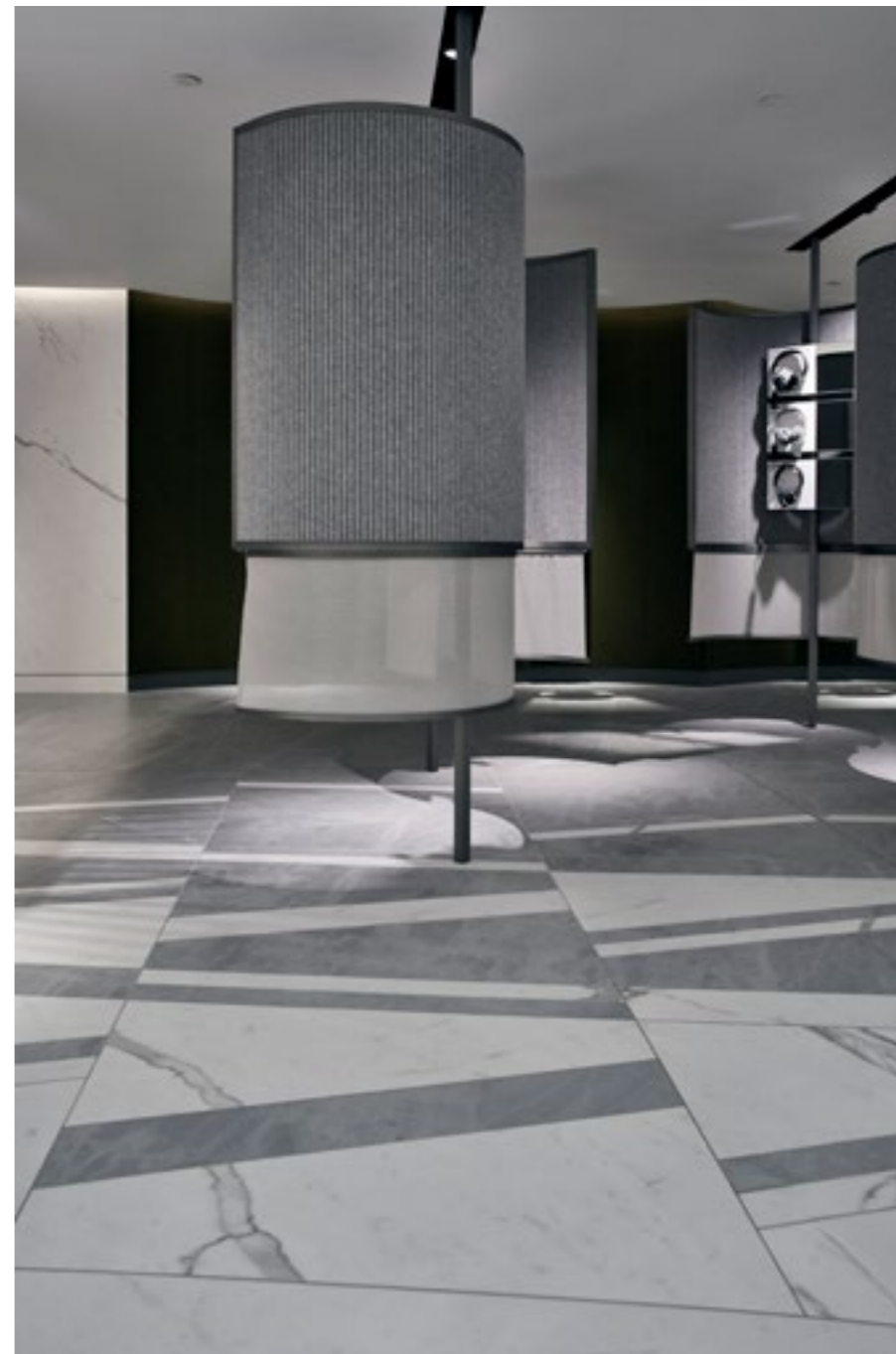
LABELLED PRECISION CUT PIECES MAKE INSTALLATION EASY (FIG.21.2)
