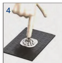
4 Firmly press the Master-Plate fastener into the adhesive until adhesive flows through the holes in the base plate.
