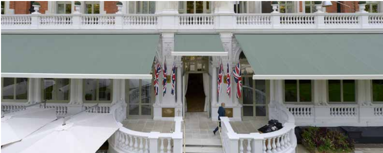
Mandarin Oriental London | UK Stylish shading. Perfectly configured to suit both the architecture and the customer's requirements.
