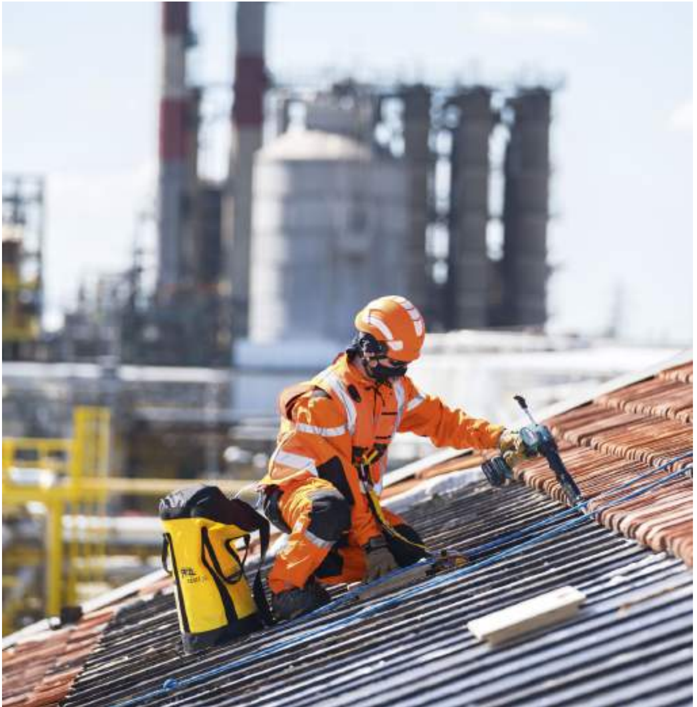
Industrial roof maintenance, Roussillon, France. © 2021 Petzl Distribution - Vuedici.org - JADE-SEQENS - Site de Roussillon
