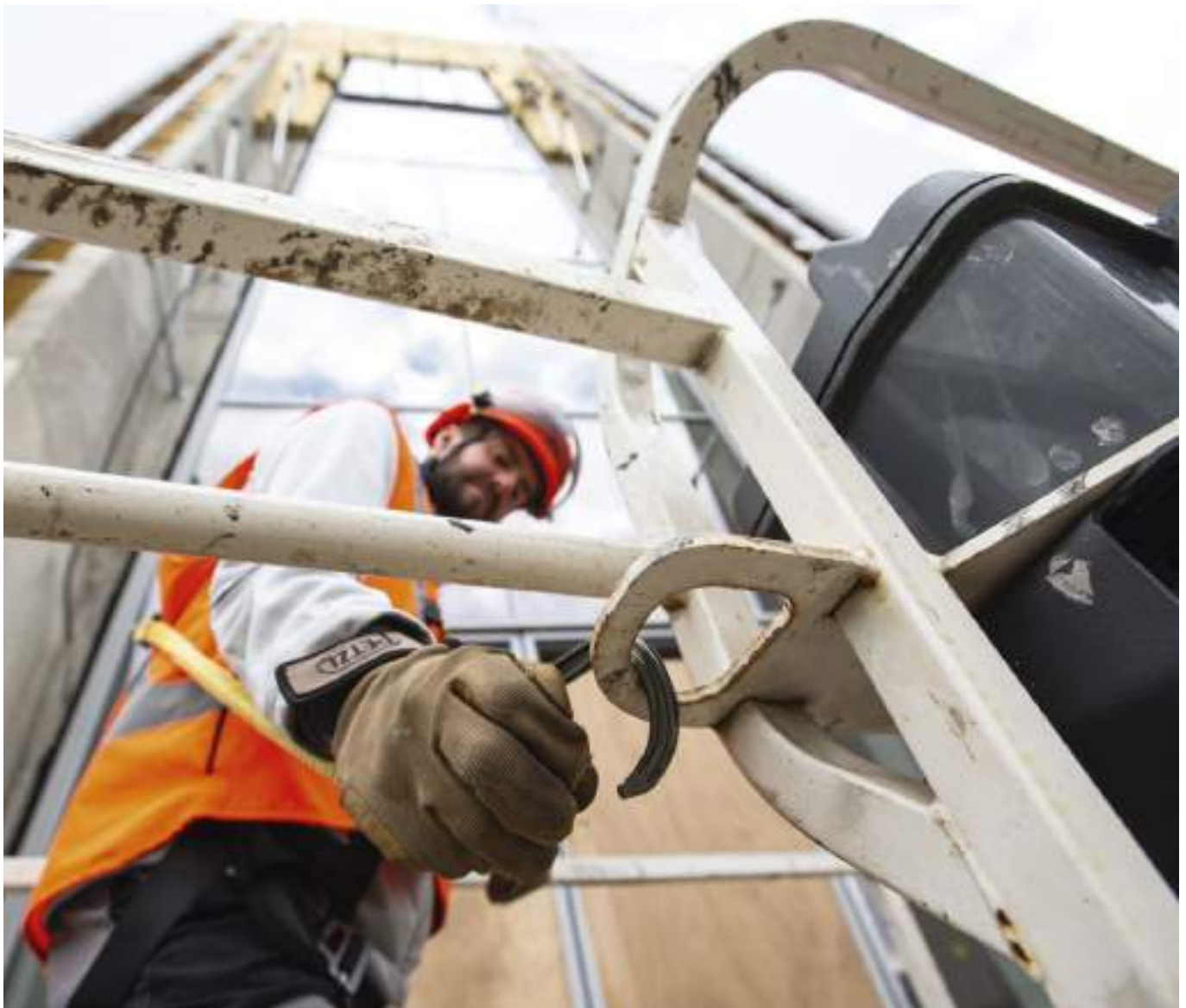
Glass window construction at the new Petzl testing facility, Crolles, France. © Petzl Distribution - Latouche
