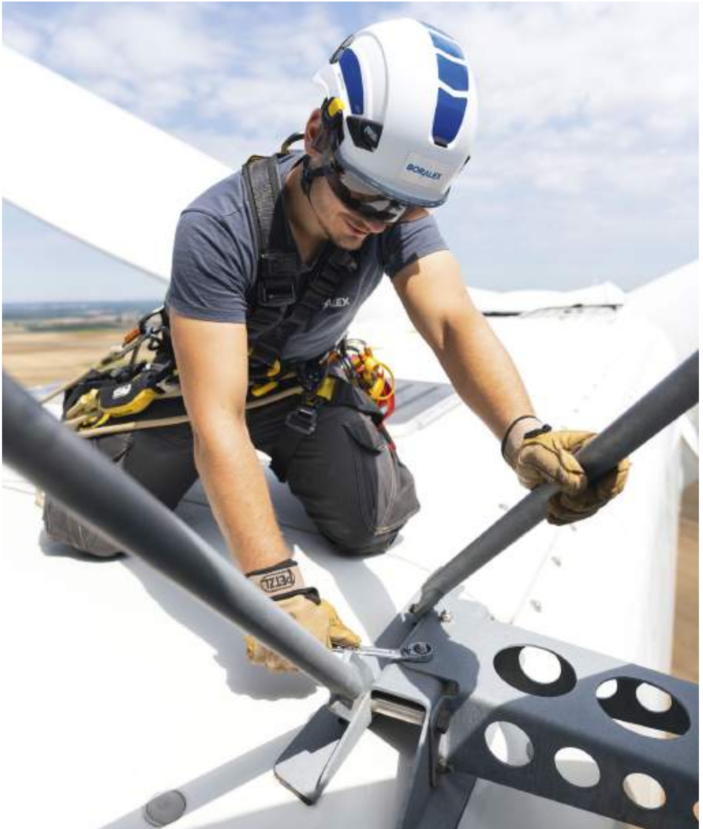
Maintenance and inspection of wind turbines in Vallée D'Arce, Champagne, France. © 2020 Petzl Distribution - Vuedici.org - Borealex SAS
