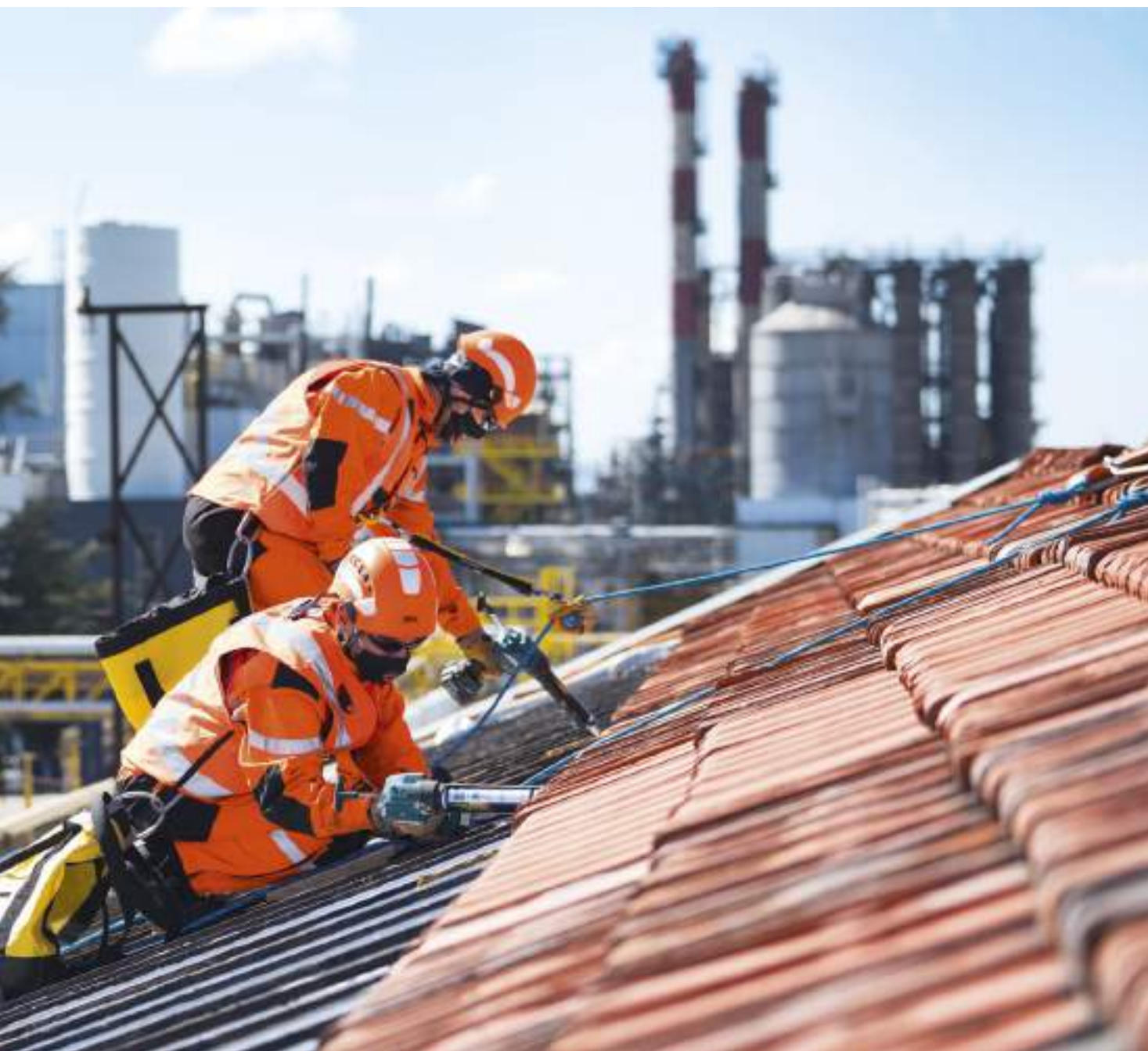
Industrial roof maintenance, Roussillon, France. © 2021 Petzl Distribution - Vuedici.org - JADE-SEGENS - Site de Roussillon
