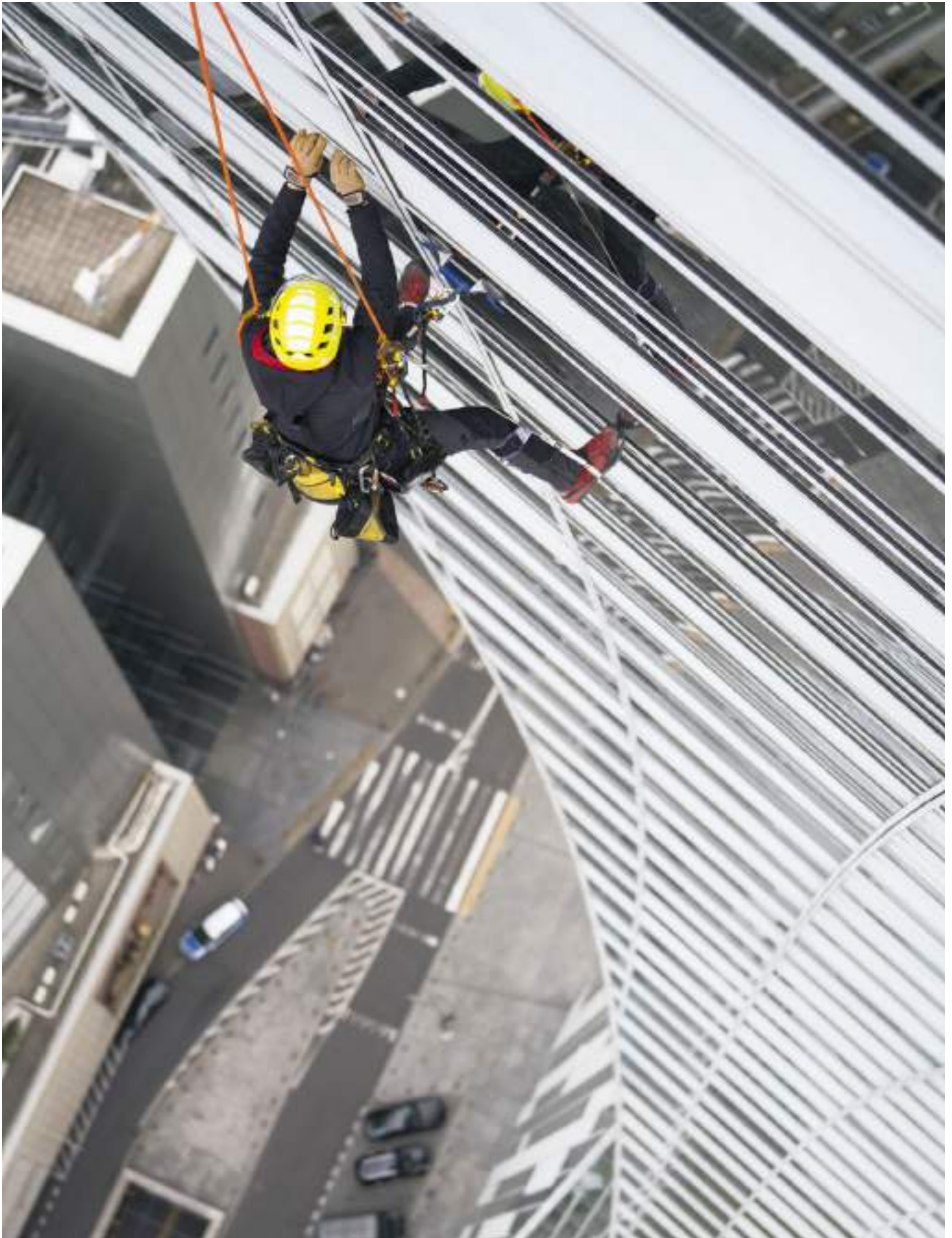
Glass panel maintenance at the Złota 44 tower, Warsaw, Poland. © 2020 Petzl Distribution - Vuedici.org - TopShell - Złota 44
