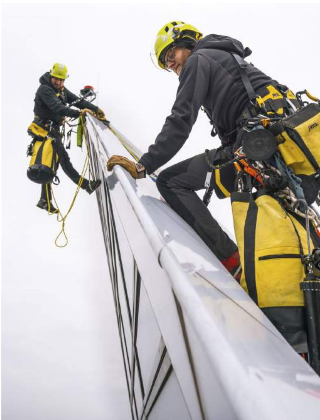
Glass panel maintenance at the Złota 44 tower, Warsaw, Poland. © 2020 Petzl Distribution - Vuedici.org - Topshelf - Złota 44
