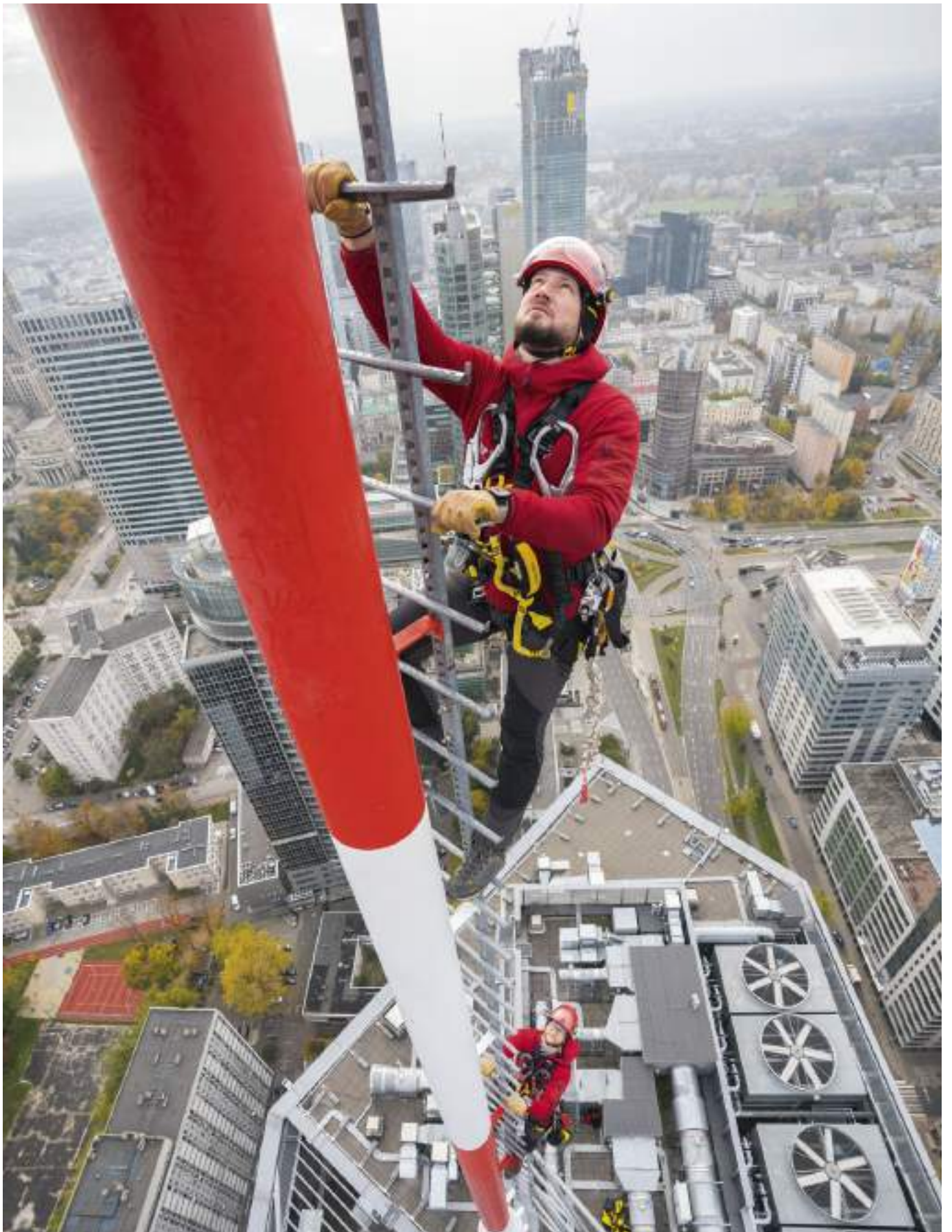
Maintenance and inspection on a telecom mast, Warsaw, Poland. © 2021 Petzl Distribution - Vuedici.org - TopSheif
