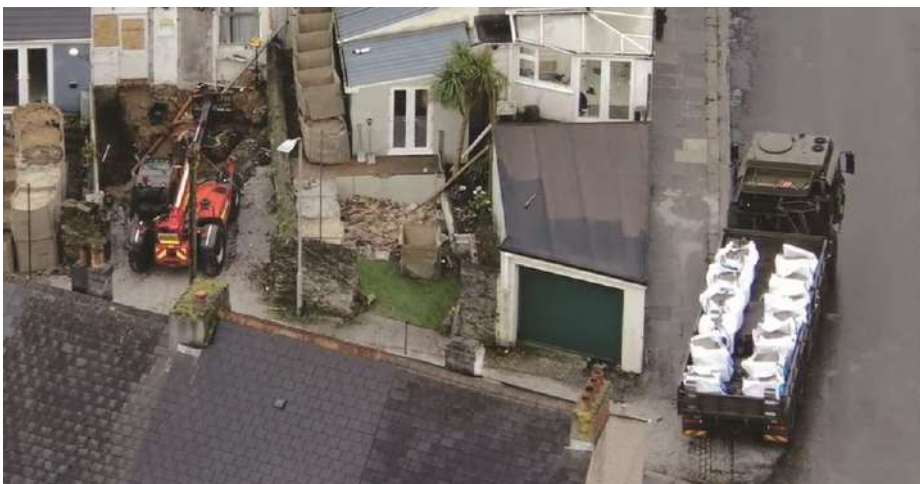
■ The truck now ready for transportation
