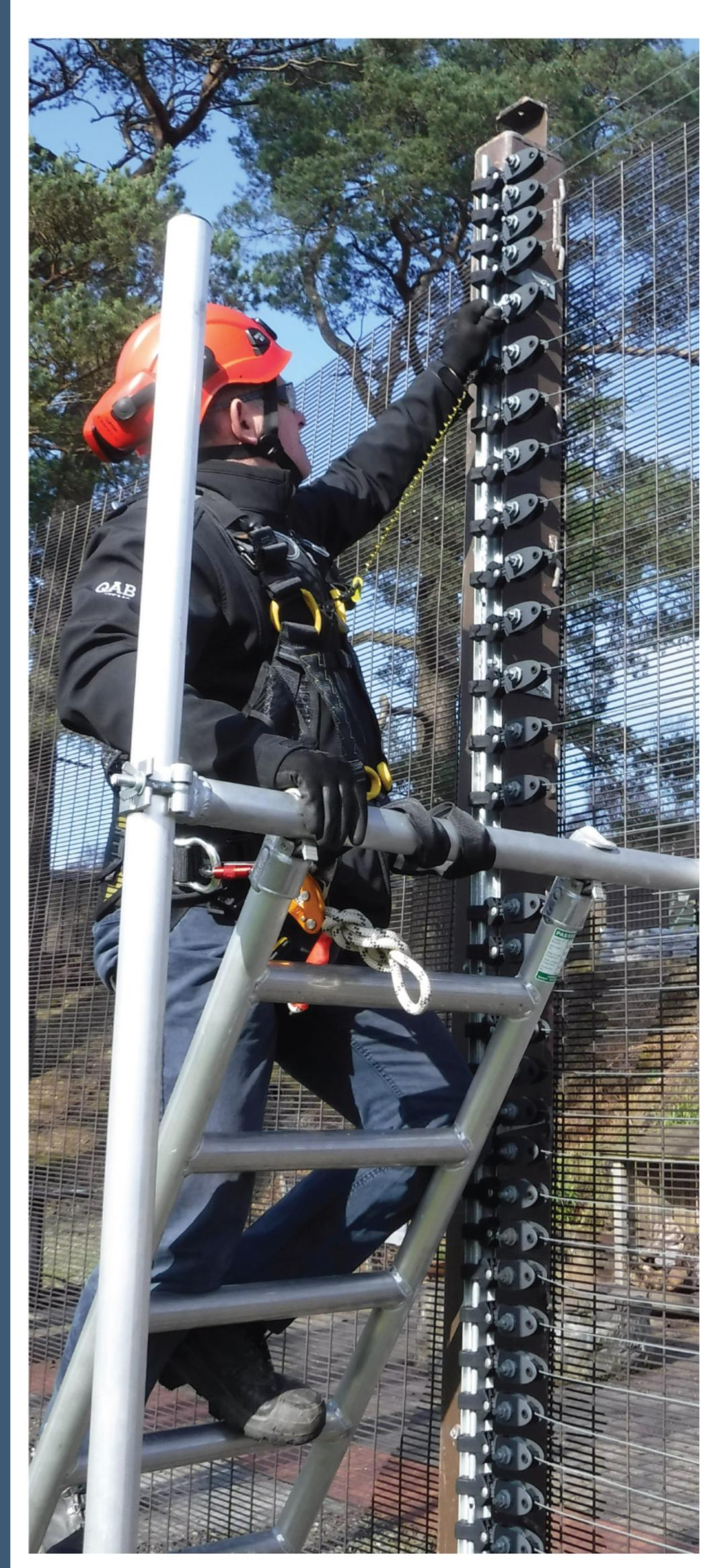
This patented system was developed by WCC Group in 2013 to allow our teams to have a safe means of access while working on security fencing.
