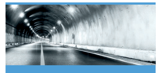
Safety for Tunnel Voice Evacuation System with Specialized Tunnel Loudspeakers
