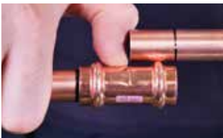
7B. Check the depth mark
