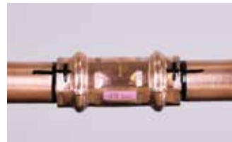
3. Mark the completed joint
