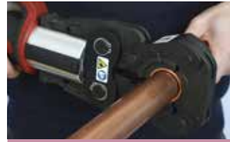
3. Complete the joint with the press tool
