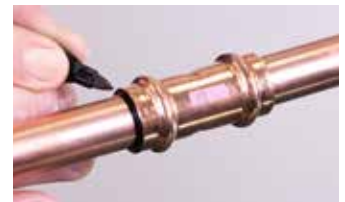
7B. Alternatively insert tube to tube stop and mark
