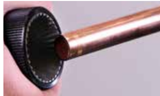
2. Deburr and remove all external sharp edges
