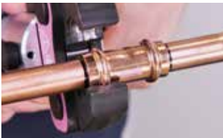
1. Align jaws squarely on the fitting
