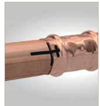
8. Mark the completed joint
