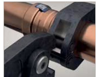
8. Engage the actuator and check insertion depth
