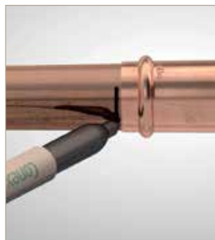
6. Assemble and mark the insertion depth
