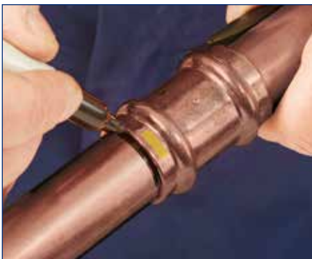
4. Assemble & mark the insertion depth
