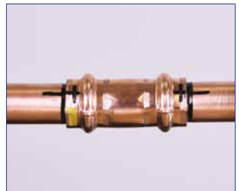
6. Mark the completed joint
