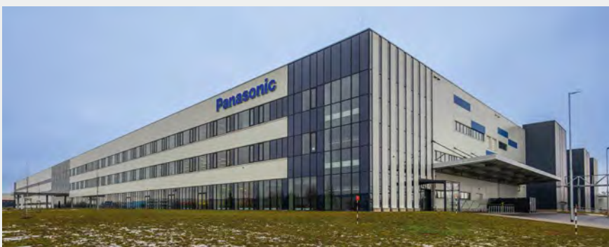
Panasonic air to water heat pumps factory. Pilsen, Czech Republic. VRF, Rooftop and Chillers.
