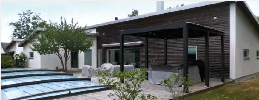
Single family house. Höllviken, Sweden. Aquarea with natural refrigerant R290.
