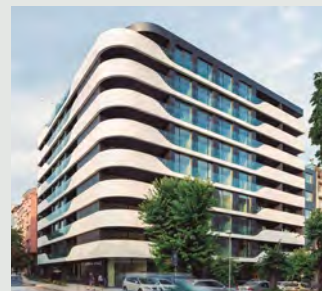
Varna Wave Building. Residential building. Varna, Bulgaria. Aquarea and Panasonic Comfort Cloud App.
