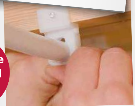
EZ Joist Clip Attach Upside Down
