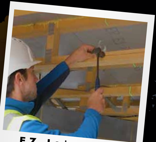
EZ Joist Clip Attach Side-on
