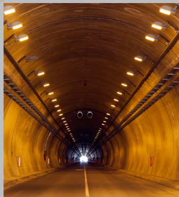
Tunnels and traffic stations
