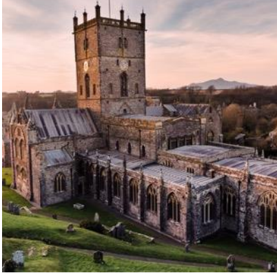
St Davids Cathedral, Pembrokeshire
