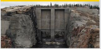
Hydroelectric concrete structures require high erosion resistance to minimize concrete wear due to aggressive water and debris. Hard-Cem fights erosion in over 6,000 m³ (212,000 ft³) of concrete structures extending the overall service life.
