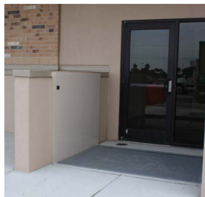
UTMB Primary Care Back Entrance, Galveston, TX
