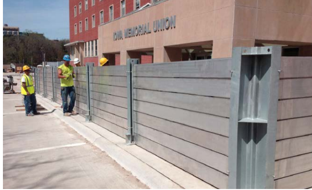
Corner Post Installation
