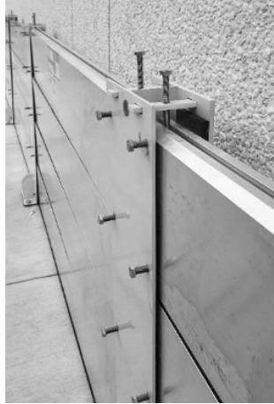
Extended Flush-Mounted Run
