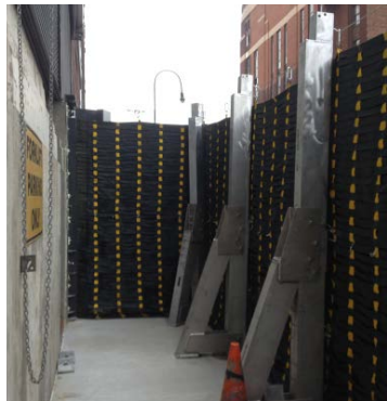
Egress Area With Support Posts
