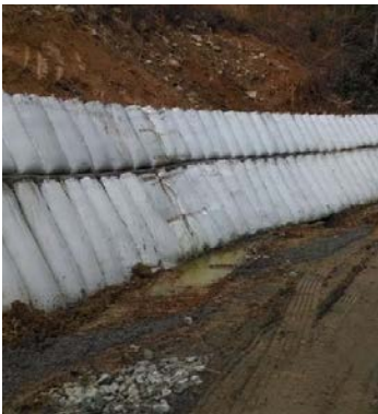
Roadside Levee Strengthening, KY
