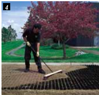
Fill rings with clean sharp concrete sand.
