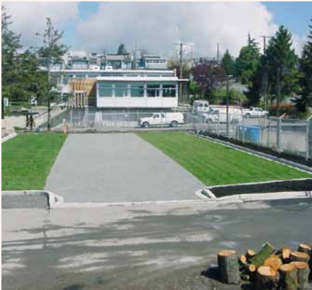
City of White Rock Operations , White Rock, British Columbia—Gravelpave 2 is used in the main drive aisle of the works yard and Grasspave 2 is used for the parking bays.
