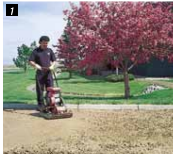
Place and compact sand and gravel road base.
