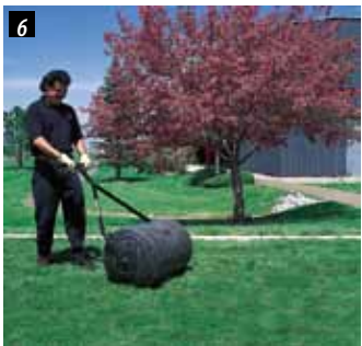
Roll sod with heavy roller.
