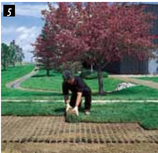
Hydroseed or lay sod.
