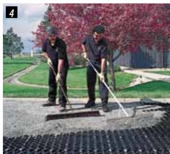
Fill rings with clean gravel.
