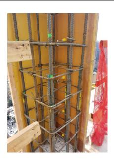
Anchor Threads installed in column forms before they close them up and pour the concrete. These will be used for leading edge protection.
