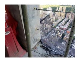
Anchor Threads installed in the column with leading edge cables attached.
