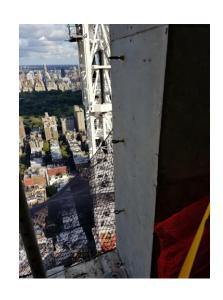
Anchor Threads installed in the column with hooks attached for leading edge cables.
