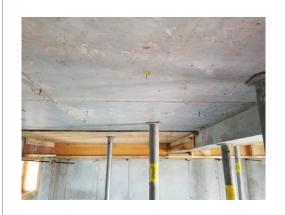
Anchor Threads installed in the deck after the pour. These Threads can be used to hang anything. No more drilling!
