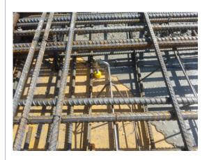
Anchor Threads installed in the deck and the pour is about to bury them in the concrete
