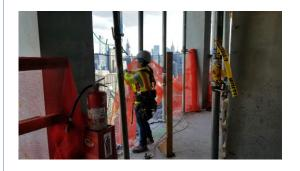
Anchor Threads installed in the column with leading edge netting attached.
